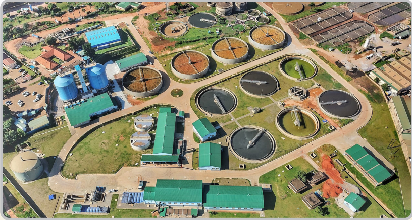
Nakivubo Wastewater Treatment Plant
